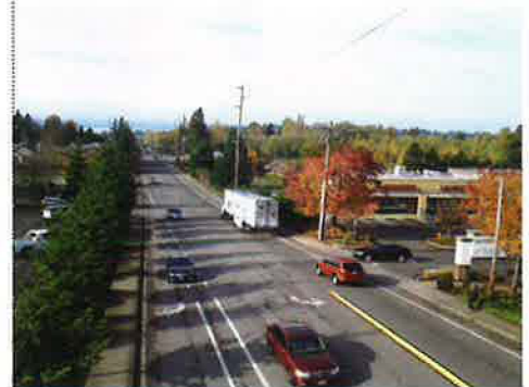
Looking West: S 216th Street near Pacific Highway - future widening into 4 lanes, a LT lane and U turn pocket. Serves shopping center (right-in/right-out)
