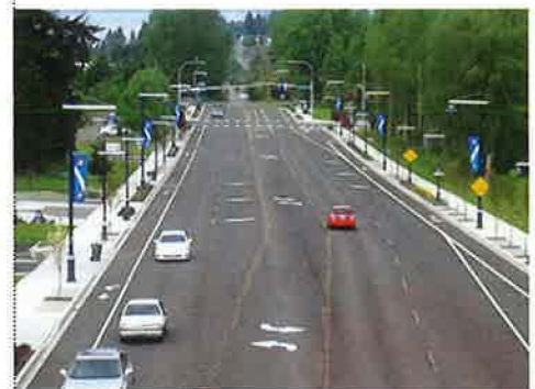
Completed S. 216th Street- East of 24th Ave S.: Similar Design Theme... 4 thru lanes plus left turn lane will match future
